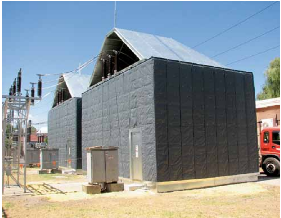
Curtains in use at the Herdsman substation.
